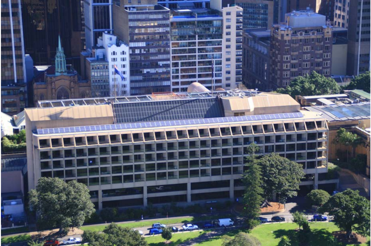
Solar Panels on Parliament House
